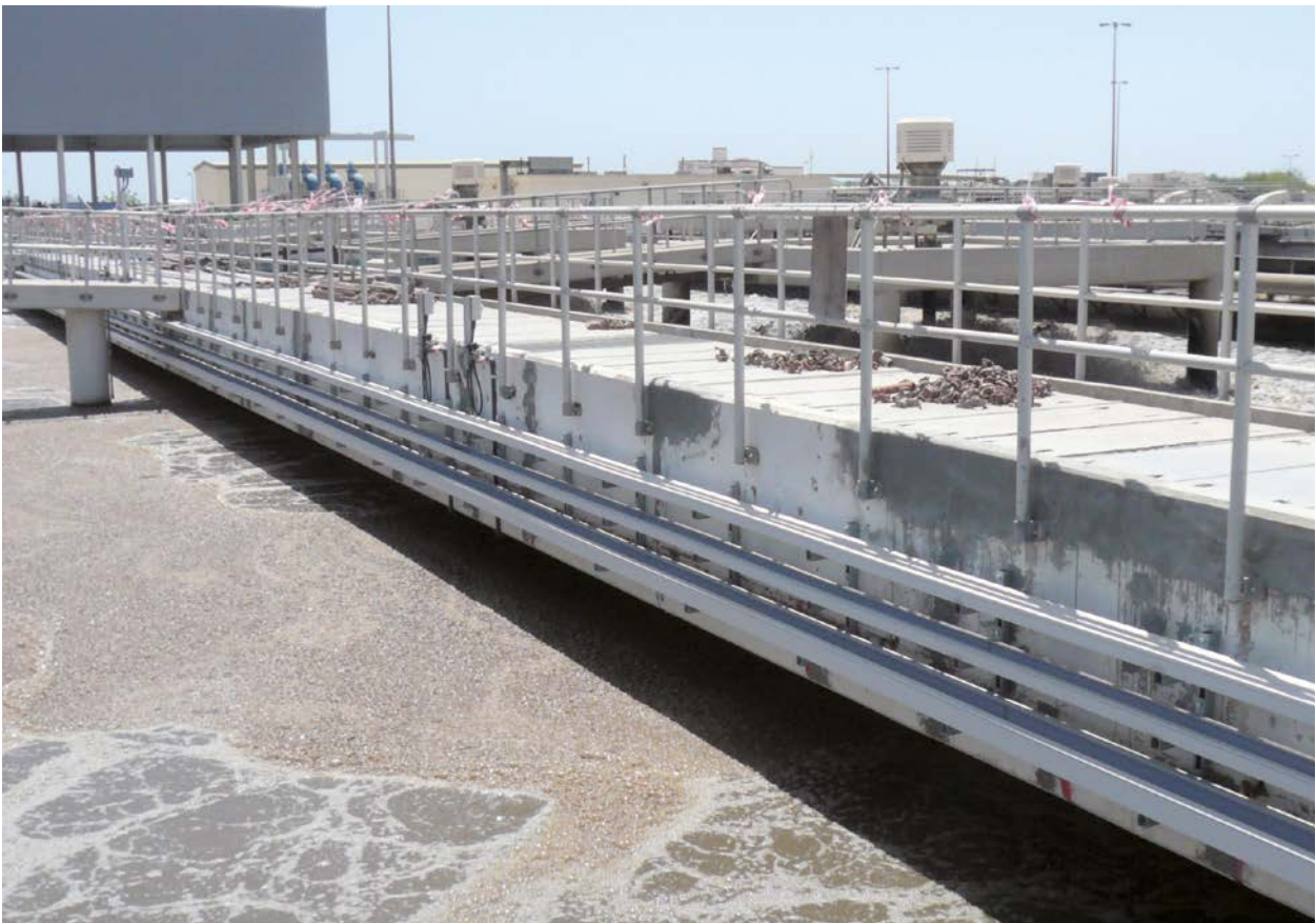
Waste water treatment plant
