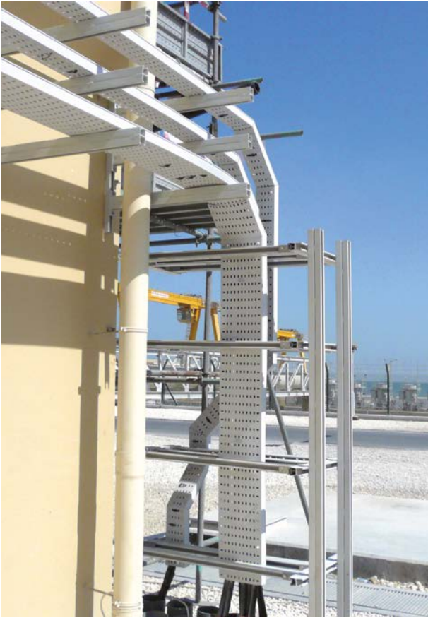
Water treatment: desalination plant
