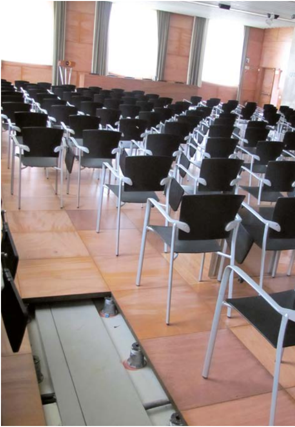
Work spaces: conference hall
